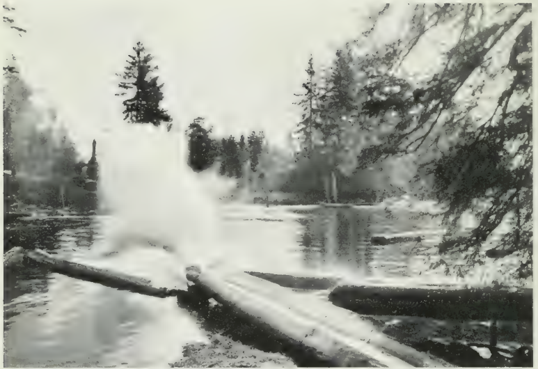
FIG. 66. TIMBER CHUTE SHOWING PROJECTING APRON : BRITISH COLUMBIA.
